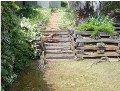
Sleeper retaining wall
